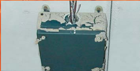
Cable junction boxes with connected cables after testing
